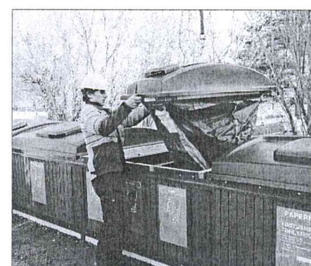
Installation of the bag+lid assembly
